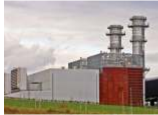
Cooling Tower Solutions
