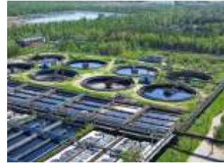
Waste Water Treatment
